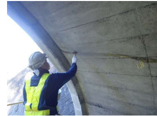
ひび割れ補修工
